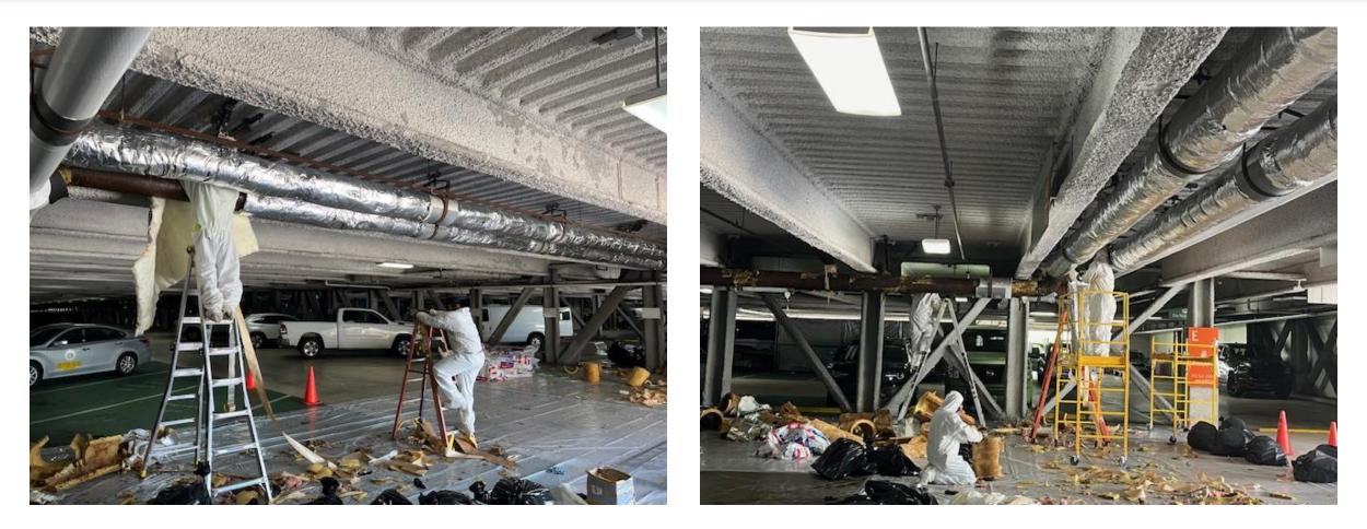
Reinsulating chill water pipes continue throughout the building. Breaks in insulation is causing leaks in the Intermediate level service corridor, Main Kitchen and Parking level.
