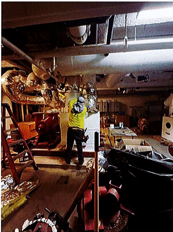
Final work on installing the pumps for the new chillers.
