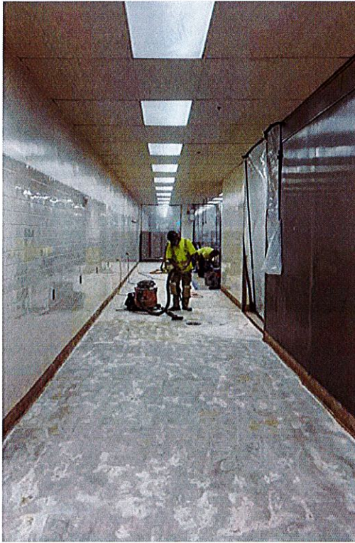
BEFORE: Prep floor and protect kitchen working areas
