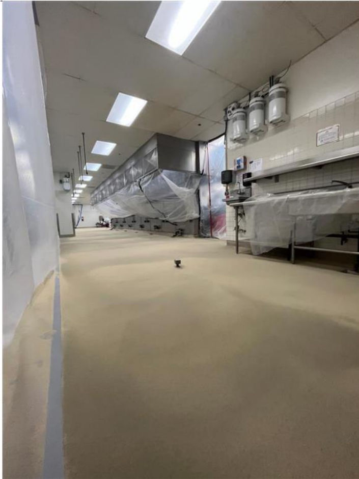
BEFORE: Old flooring
