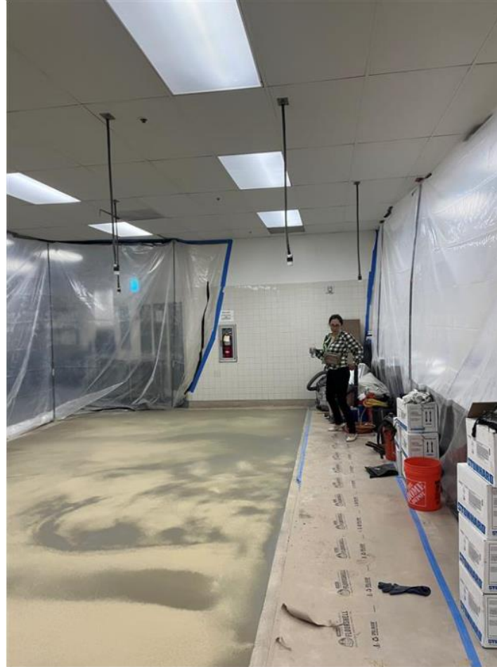
REMOVAL: Flooring preparation
