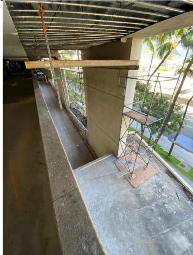
Scaffolding was erected over the Parking entrance ramp for safety and to facilitate work on the Kalakaua planters.
