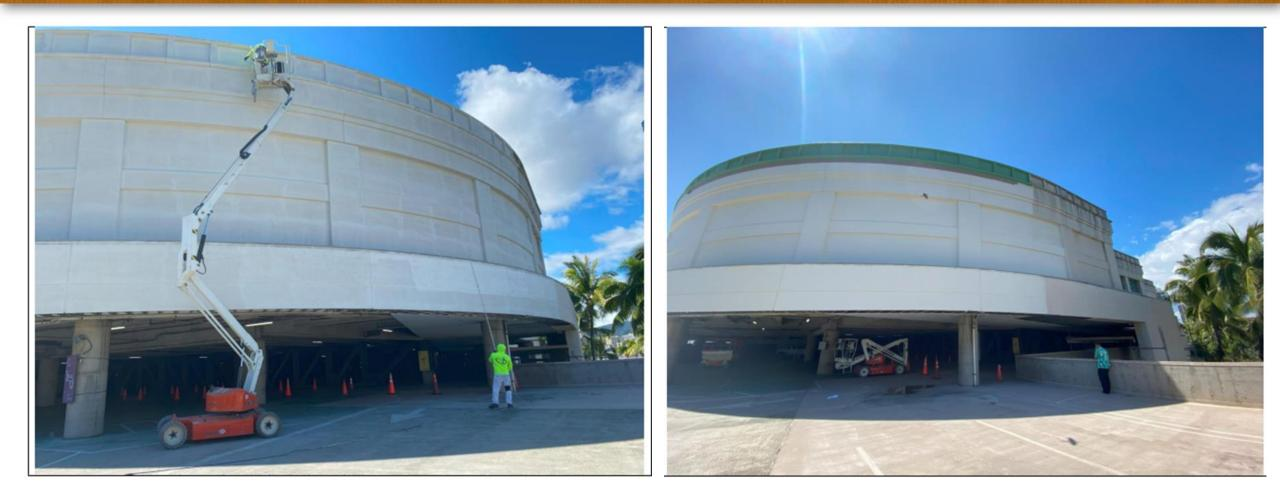
Painters working on the curve around Theatre 310. The Parking deck provides easy access using the boom lifts. Other areas are challenging requiring scaffolding and swing stages.
