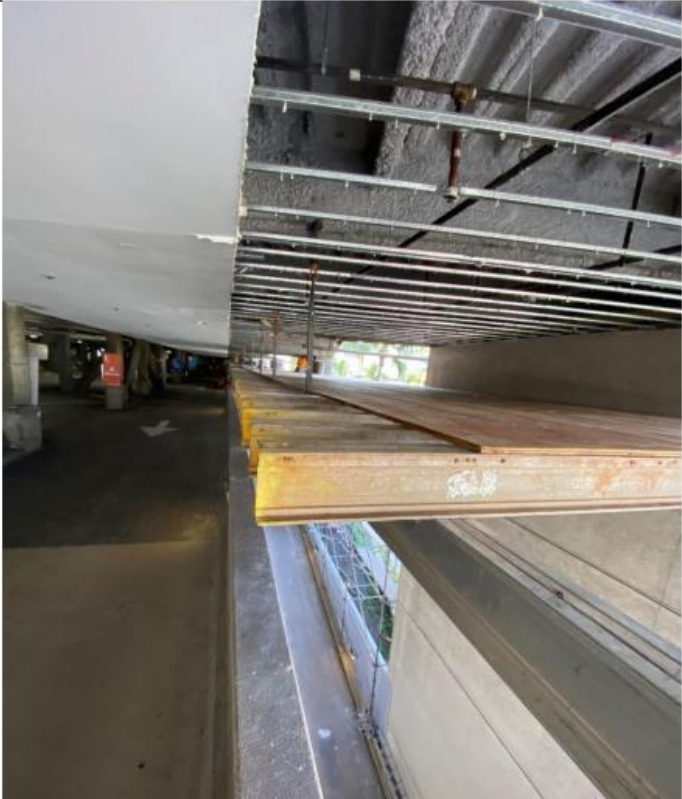
Scaffolding was erected over the Parking entrance ramp for safety and to facilitate work on the Kalakaua planters.
